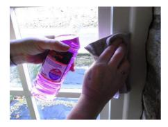
Clean your window frame surfaces, onto which you will be attaching the panel using methylated spirits or a similar degreaser.
